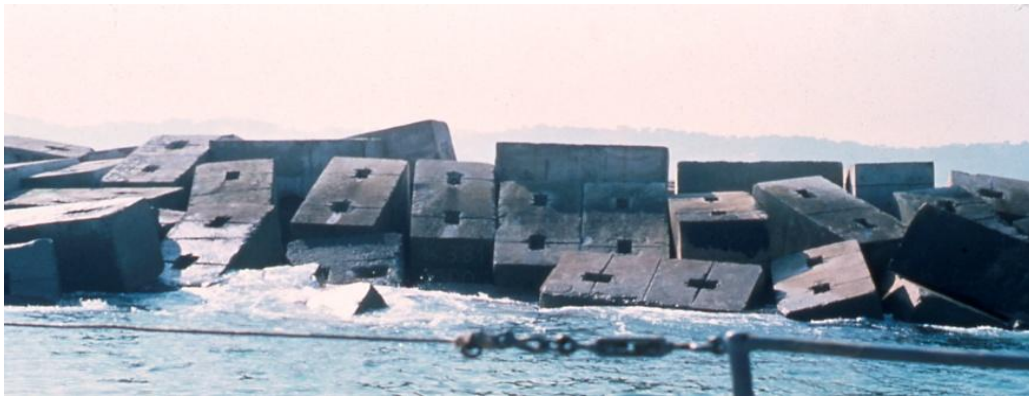
Figure 1 Example of breakwater built in the 1930'ies and armoured with large rectangular blocks.
