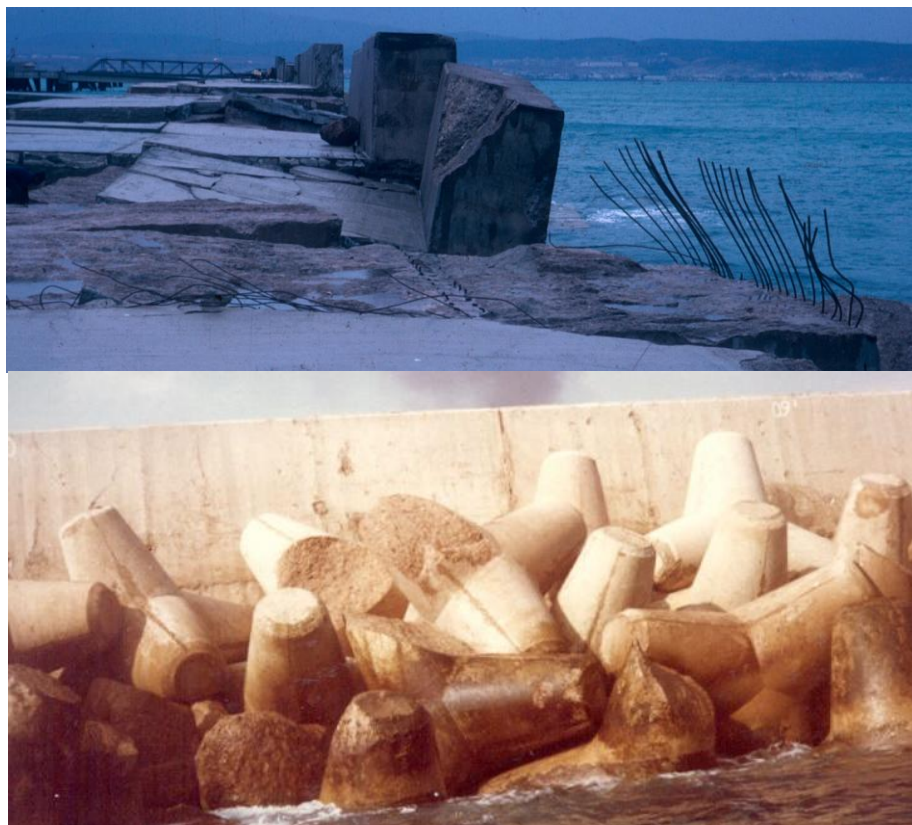
Figure 6 Photos of Arzew el Djedid breakwater damage. Above, most damaged sections and below, section with settlement of entire armour layer and broken units.
