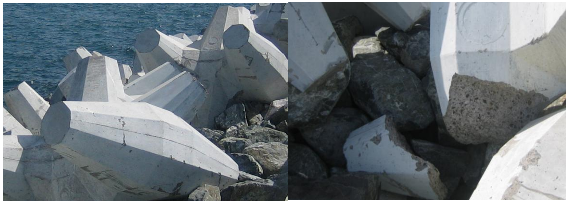
Figure 14 Example 2: Core-Loc breakwater with approx. K_D=16 . Note settlement of entire armour layer creating gap at wave wall and some breakage.
