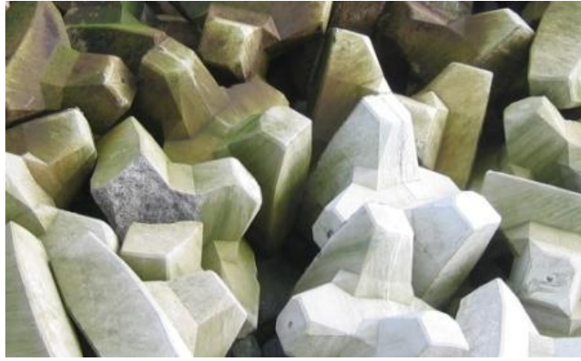
Figure 13 Example 1: Accropode breakwater with approx. K_D=15 after exposure to design event. Note broken units and openings, non-interlocking units.
