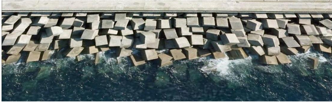
Figure 8 The armour layer on the Bilbao Breakwater 2013 (Google Earth).
