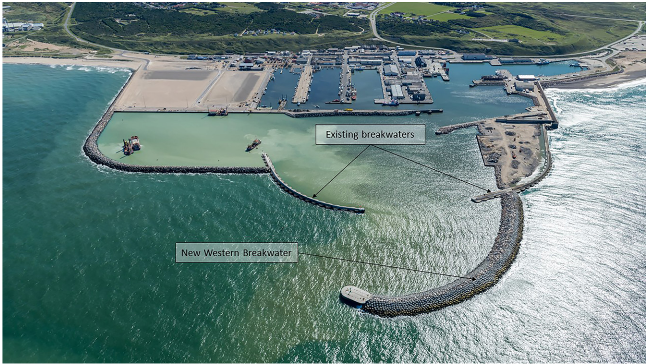
Figure 2. Port expansion project
