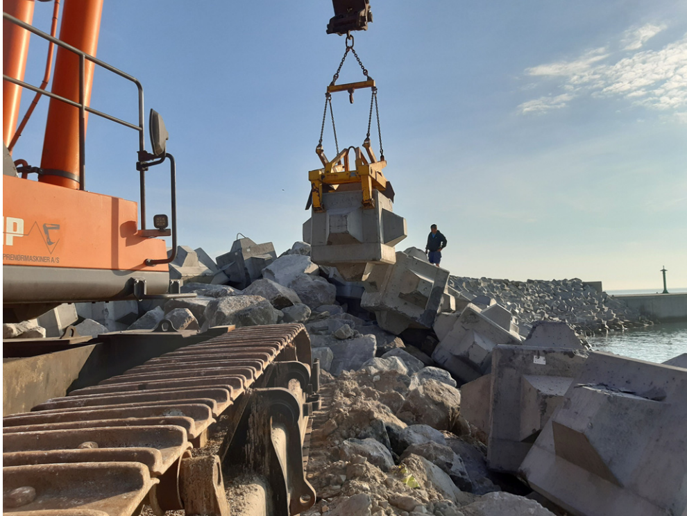
Figure 15. Placement of Cubipods with free-hanging lifting tool
