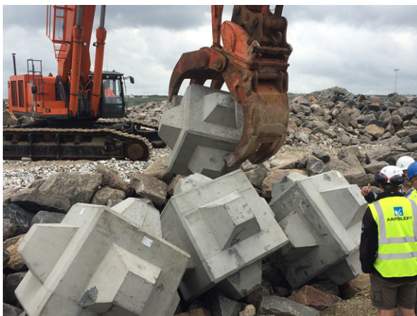
Figure 16. (Left) Excavator equipped with special designed grab. (Right) 30 t Cubipod with wire grommet
